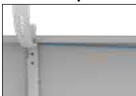
Put a string between the high and low bracket. It will help you to place the other brackets.
